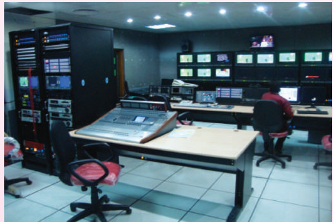
New Studio of Bangladesh TV Completed and handed over to BECIL
